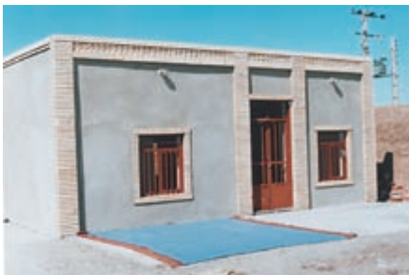
Fig 10: New reconstructed houses in Bam after less than two years
