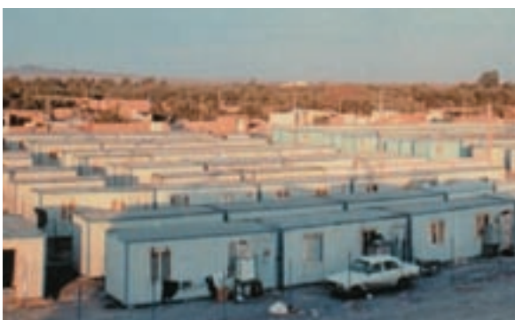
Fig 6: Temporary shelters in plot of lands (top) and pre-fabricated camp cities (bottom)
