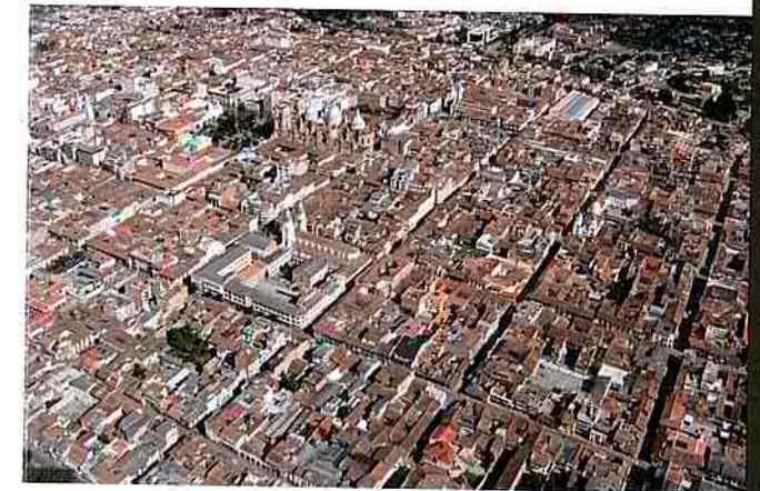
WH Site Historic city of Cuenca (Ecuador) – focus area of maintenance plan in preparation by Universidad de Cuenca and the K.U. Leuven.
